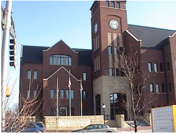
New Arlington Heights Municipal Center kitty corner
